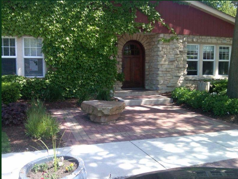
Street view of office at 126 S. Main Street in Oswego
